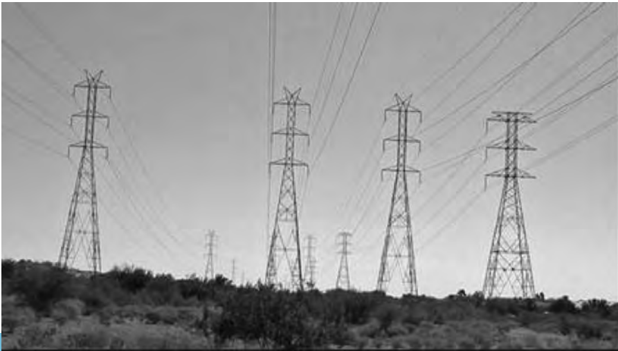
FIGURE 19.3 Transmission line corridor.
